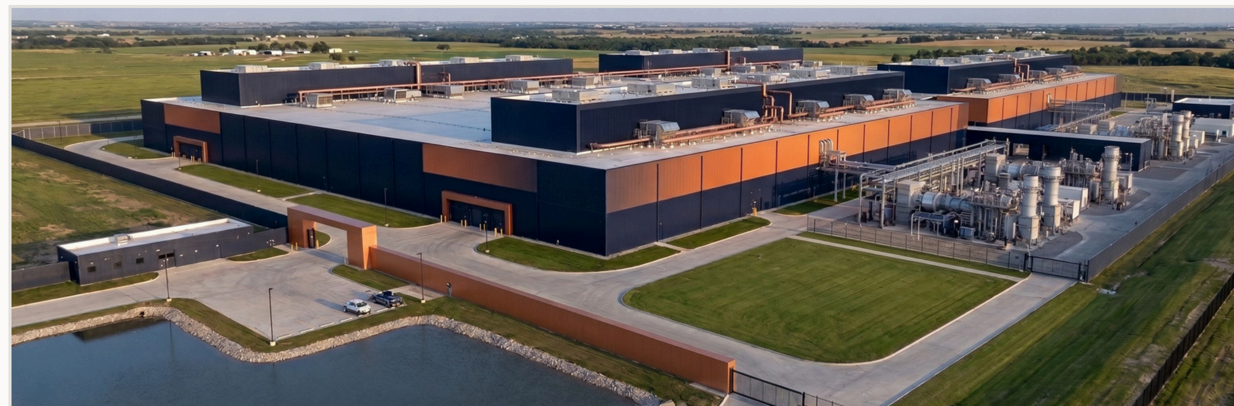
A modern data center campus. Low-profile buildings, on-site power equipment, screening and stormwater management.
